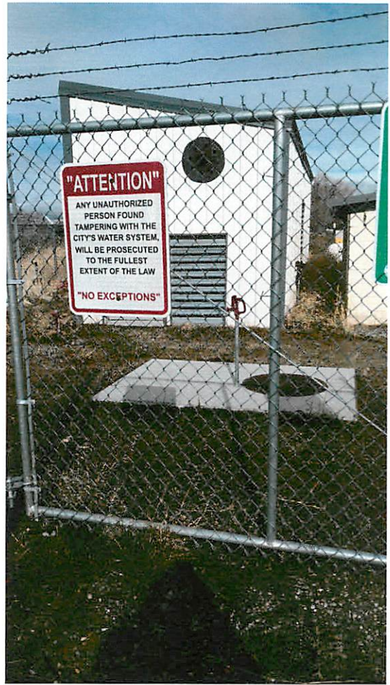
Gated generator house
