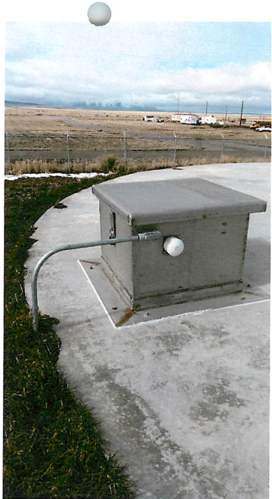
Manhole of storage tank
